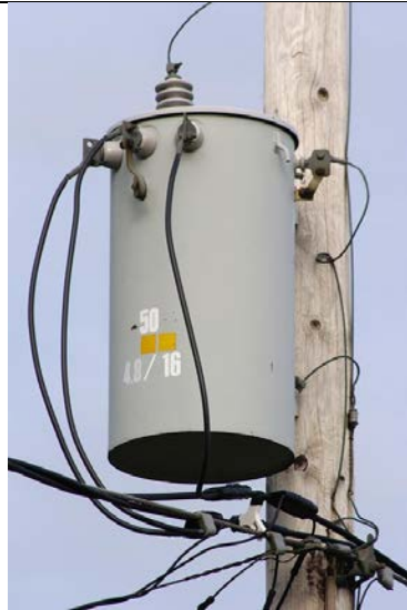
Distribution Transformer providing L-N-L single phase 120/240V service (aka split phase) (above). Diagram (below) 323
